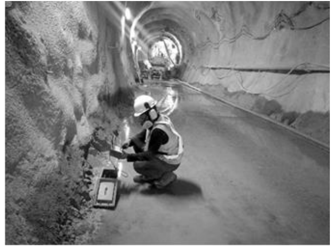
Figure 11: Instalation and check to an seismograph parameters before a blast.
