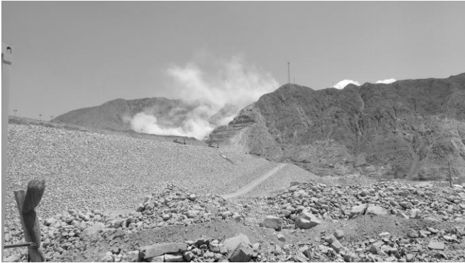
Figure 1: Dam Palo Redondo (May - 2016)
