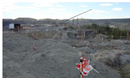
Figure 17: Covering the blast area with sand, craning to avoid damaging EDD cables
