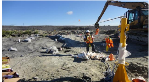
Figure 16 : Drilling (right) and loading hole (left) safely over an instable area
