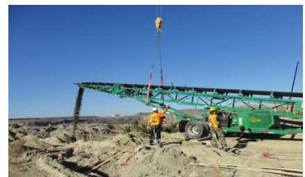
Figure 17: Covering the blast area with sand, craning to avoid damaging EDD cables
