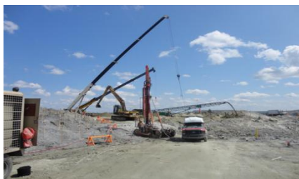
Figure 17: Covering the blast area with sand, craning to avoid damaging EDD cables
