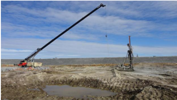
Figure 16 : Drilling (right) and loading hole (left) safely over an instable area
