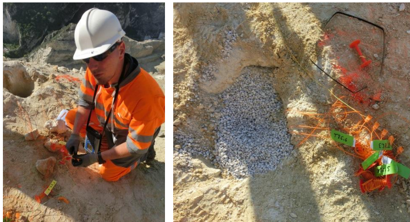
Figure 16. Programming the electronic detonators
