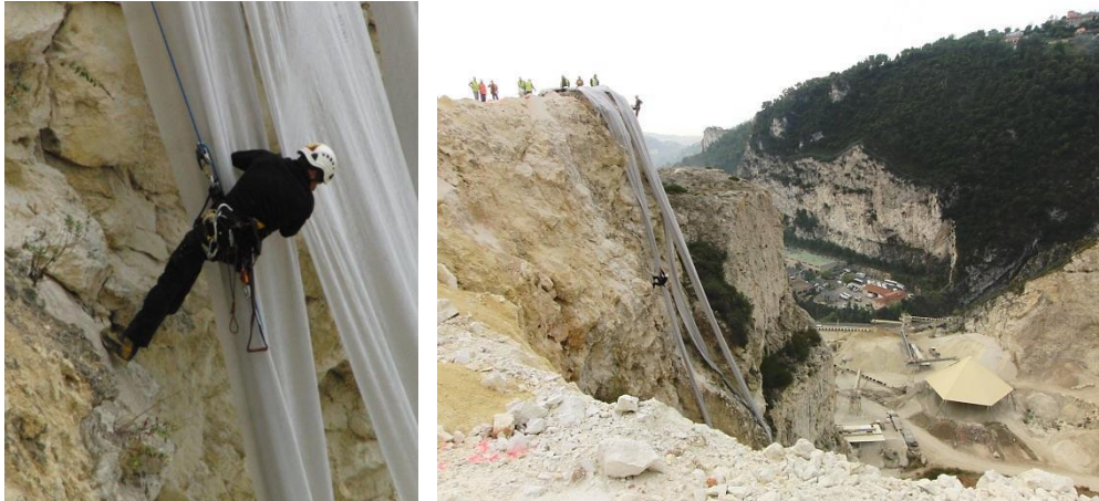
Figure 67. Installing the protection on the free face
