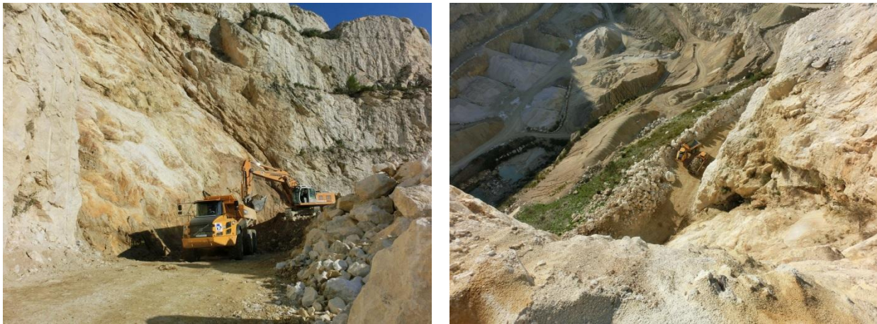
Figure 13. Bottom and top view of the rock barrier being implemented
